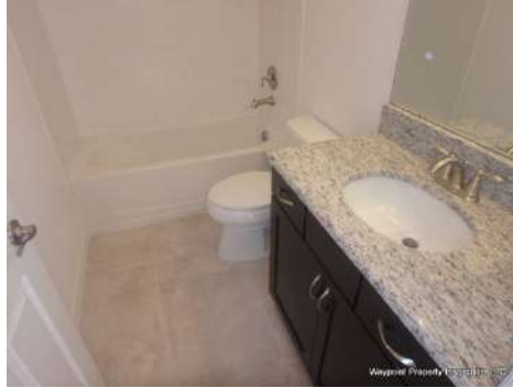
Hallway bathroom (front).
