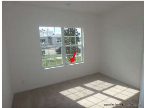
The interior and exterior of the windows should be sealed at various areas.
