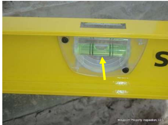
Concrete form measured level at various areas
