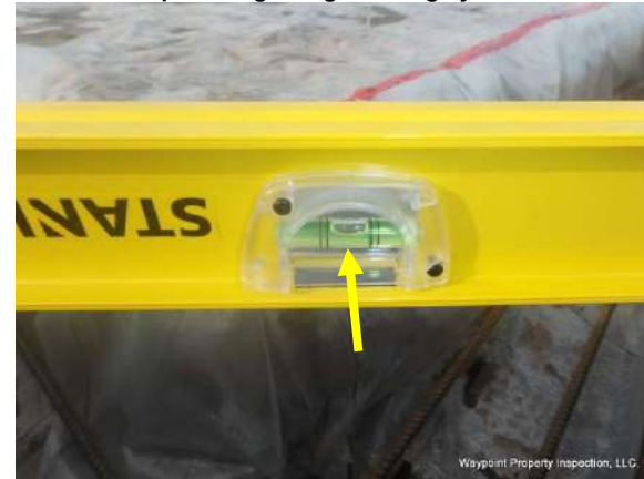
Concrete form measured level at various areas
