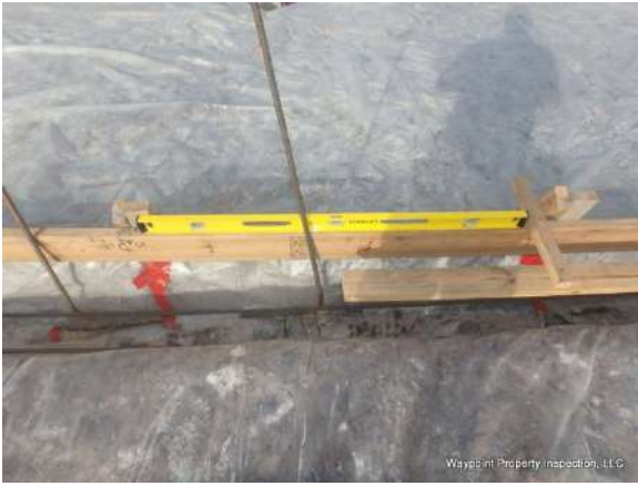
Concrete form measured level at various areas
