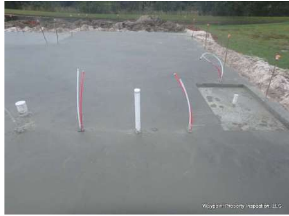
Bathroom Plumbing Penetrations
