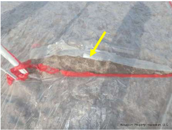
Vapor barrier had visible gaps that should be sealed.
