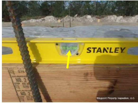
Concrete form measured level at various areas
