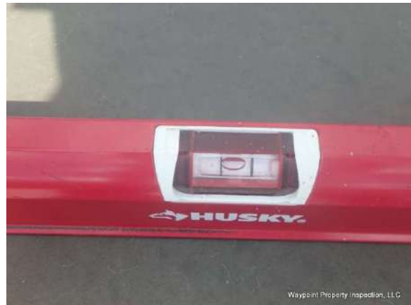
Garage had proper slight pitch toward the door area
