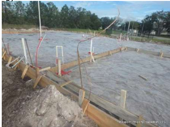
Laundry plumbing including water softener line / Water heater plumbing and grounding system.
