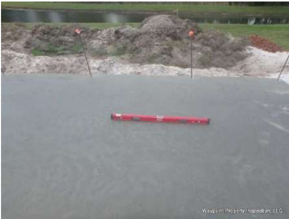
Foundation measured level at various areas.
