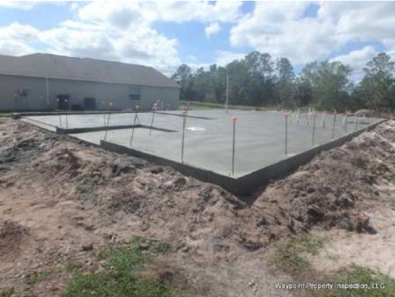
Front / Right front corner
