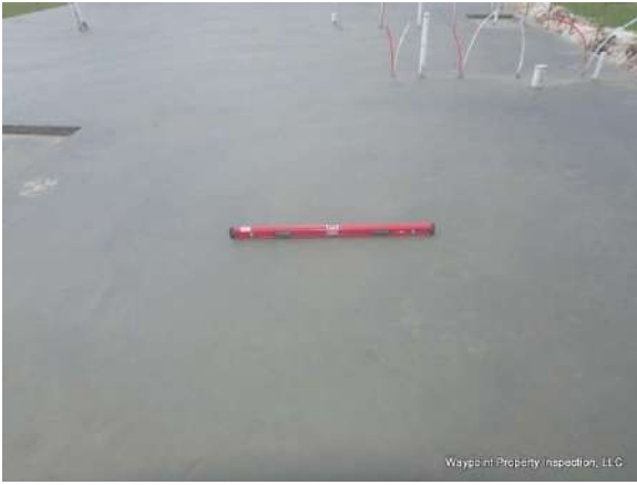
Foundation measured level at various areas.
