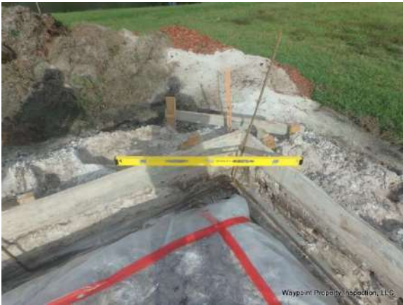
Concrete form measured level at various areas
