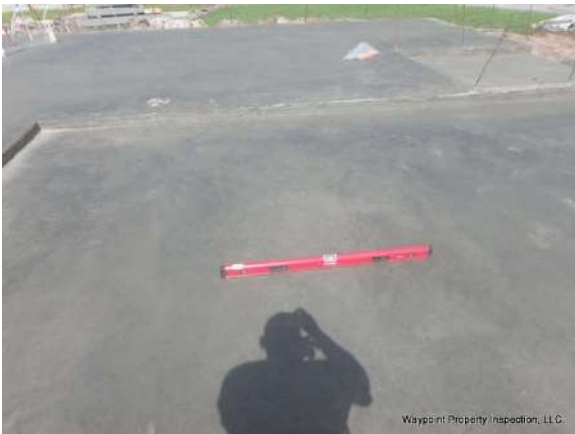
Garage had proper slight pitch toward the door area
