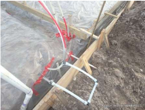
Laundry plumbing including water softener line / Water heater plumbing and grounding system.
