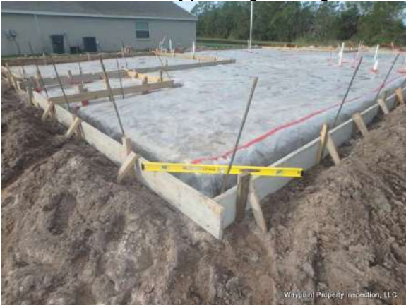
Concrete form measured level at various areas
